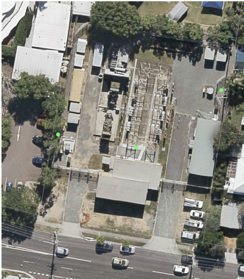
Figure 3: Chermside Substation (geographic view)
