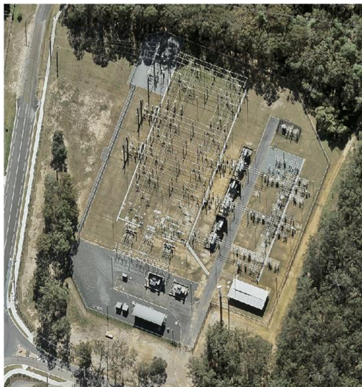
Figure 3: Caboolture Substation (geographic view)
